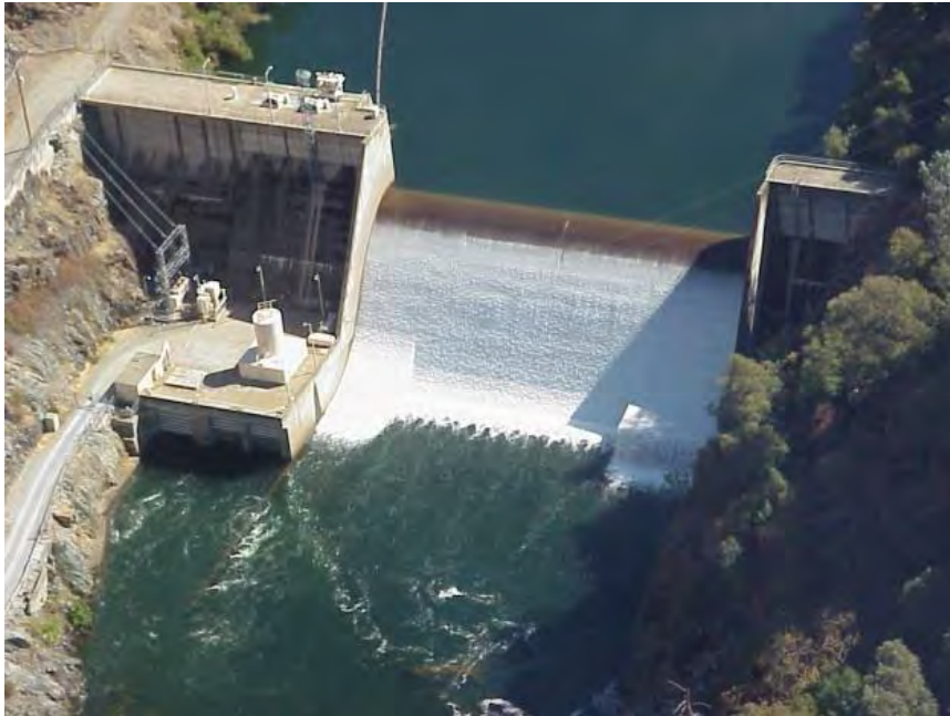
Chili Bar Dam, Photo Credit: PG&E
